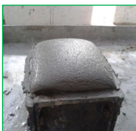
Aerated Geopolymer concrete
